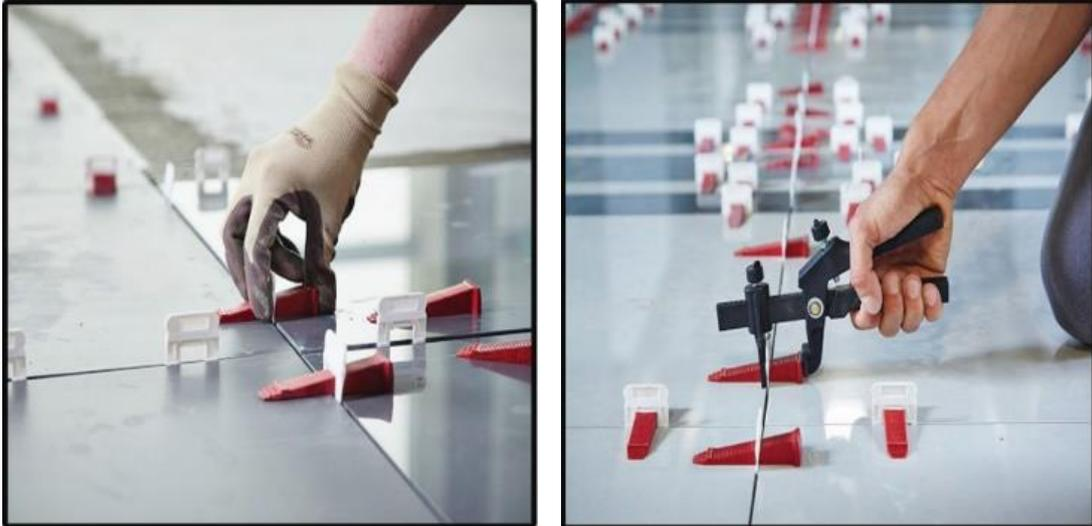
4- Finally, to remove the clips and wedges, gently tap the clip in the direction of the ceramic tile joints with your safety shoes or with a plastic hammer so that the lower part of the clip remains under the ceramic tile and the upper part and the wedge come out. This should be done when the adhesive under the ceramic has dried and the ceramic tiles do not move due to the tapping.
