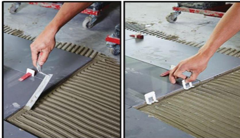
2- Then place the next ceramic tile on the other edge of the clip and adjust it by a rubber hammer.
